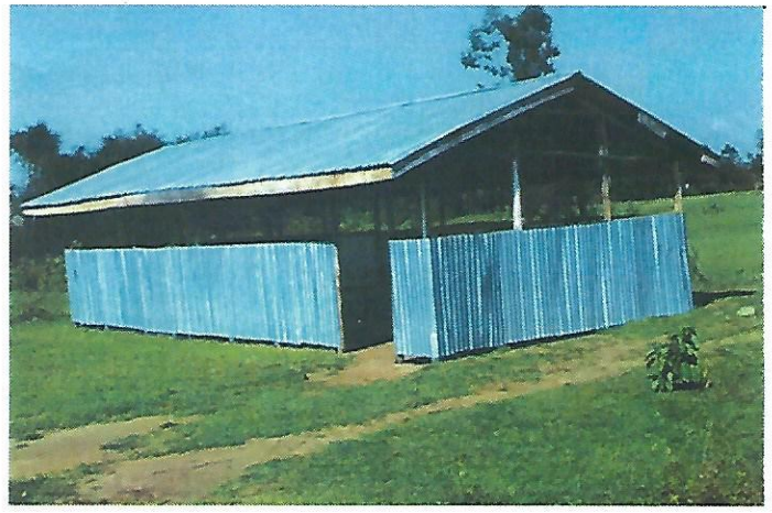
New chicken house under construction by Pastor Joseph Allen
