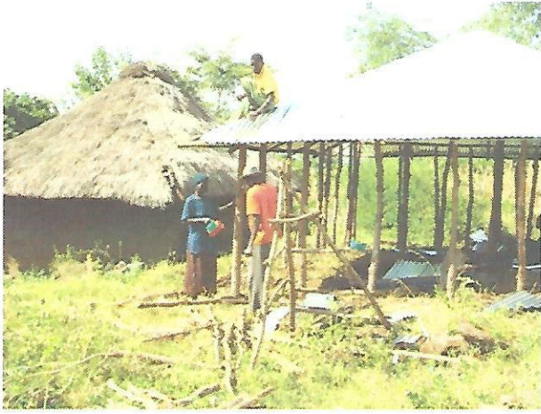
Typical mud hut construction
